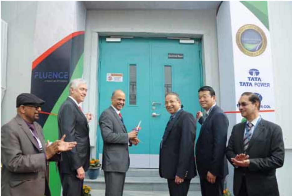
The 10 MW grid connected battery system at Tata Power's Delhi substation uses Advancion energy storage platform from Fluence.
