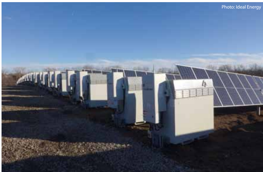
NX Flow vanadium redox flow batteries connected to a solar array.
