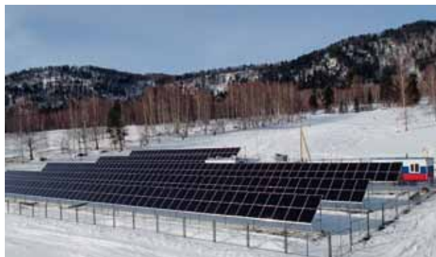
Pictured: A 100 kW off-grid solar-diesel power generating system in a remote village in Altai, Russia.
