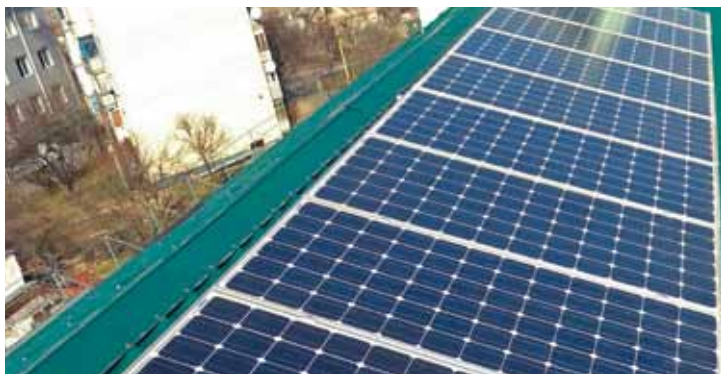
Rooftop solar is a new trend in Ukraine. This 9 kW system is installed on top of an apartment block in Kherson, southern Ukraine.
