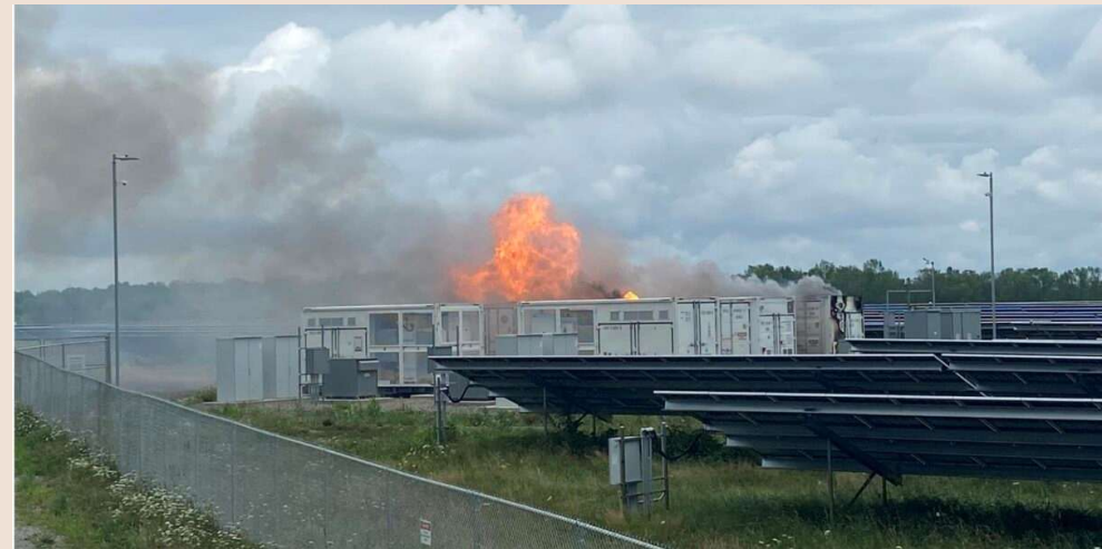
BESS-Brand Chaumont Solar Farm, New York, USA Quelle: PV Magazin
